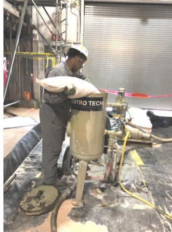
Loading batches of SENTROMAX™ dry chemicals into SENTRO's blasting machine.
