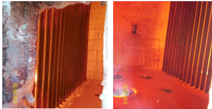
After cleaning: Tubes are clean; refractory (ceramic fiber) is undamaged
